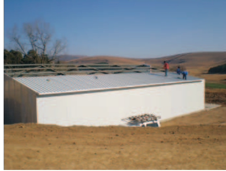
Construction of large Cold Room for Potato Storage
